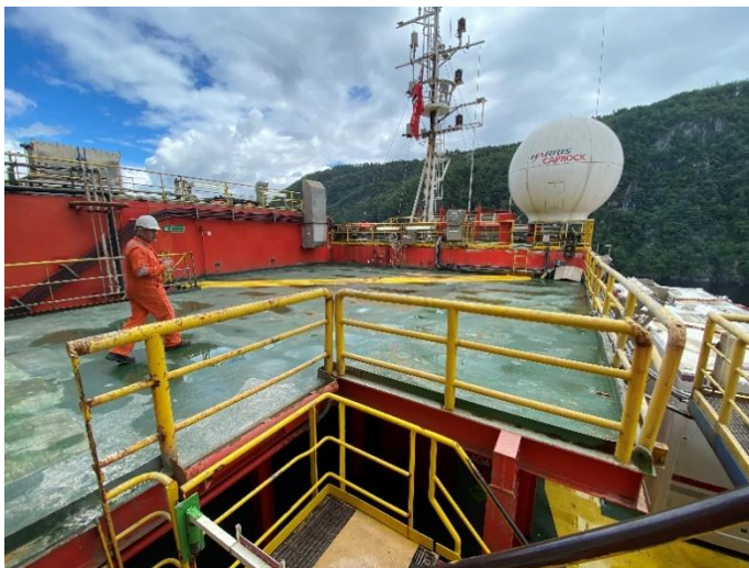
Figure 0-44: Wireline unit area
