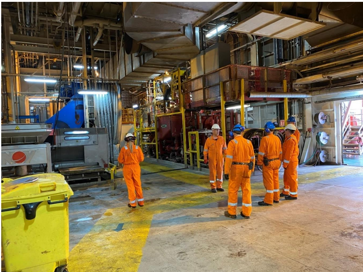
Figure 0-14: Sack store and mud pump room.
