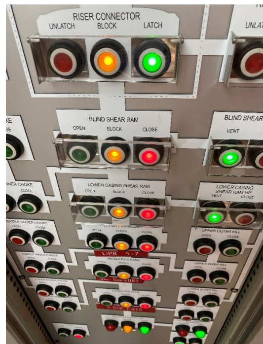
Figure 0-21: Mud mixing & high-pressure mud system schematics (left) and BOP Control panel (right)
